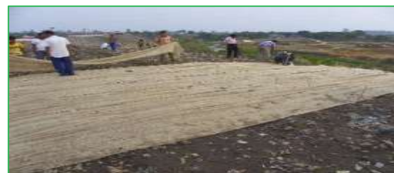
Covering of surface with Jute & other capping Material
