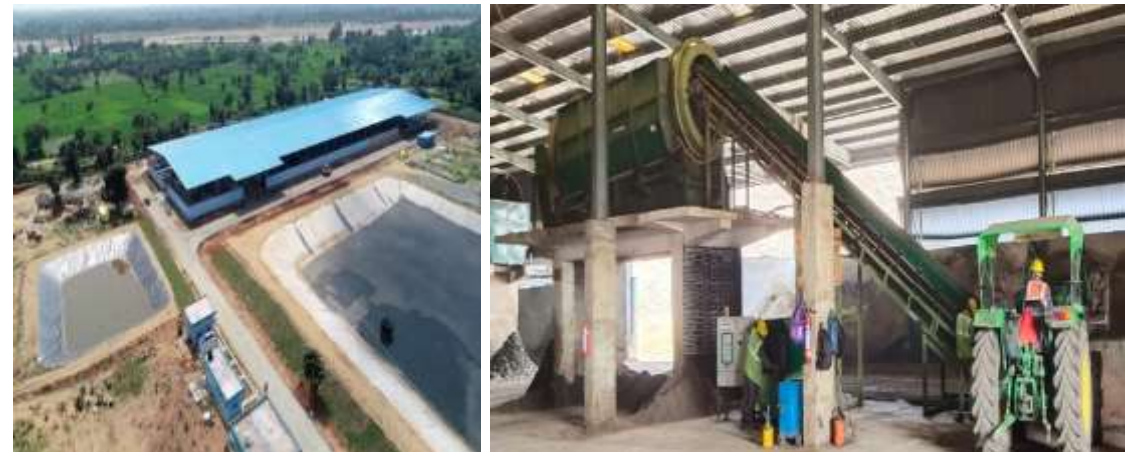
Kachhar Integrated Solid Waste management Facility (Bilaspur)
