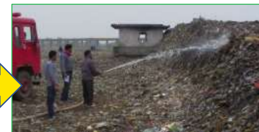
Sprinkling of water for compressing the heap
