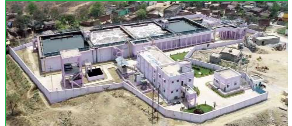
Raigarh (Banjipali): 25 MLD
