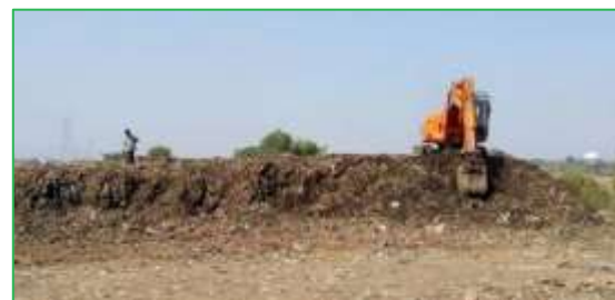
Formation of garbage heap and primary segregation
